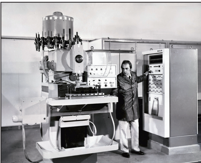
The FUW C 450 NC machining centre with contouring control
